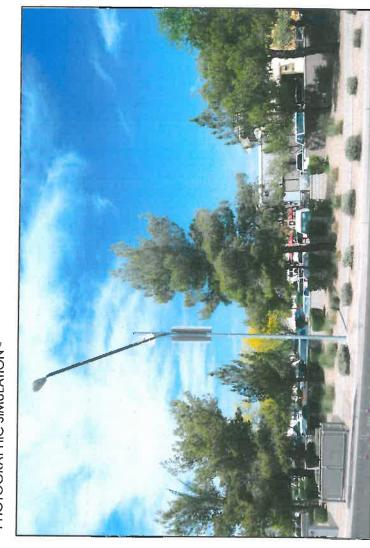
PROPOSED INSTALLATION OF LESSEE ANTENNA ARRAY AND MICROWAVE DISH MOUNTED TO 29' REPLACEMENT UTILITY POLE. ADDITION OF LOW-PROFILE SUNWEST EQUIPMENT CABINET, WITH PERFORATED SHEET METAL SCREENING.
